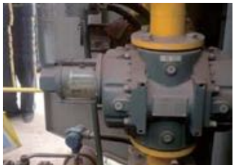
Gas roots flowmeter in gas mixture field
