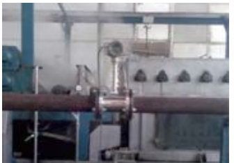
Vortex flowmeter in boiler system for steam measurement
