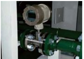
Liquid turbine flowmeter in water supply plant
