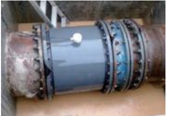
Magnetic flowmeter in under well field
