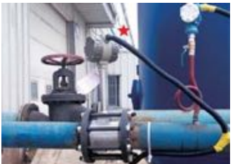
Vortex flowmeter in oxygen measurement
